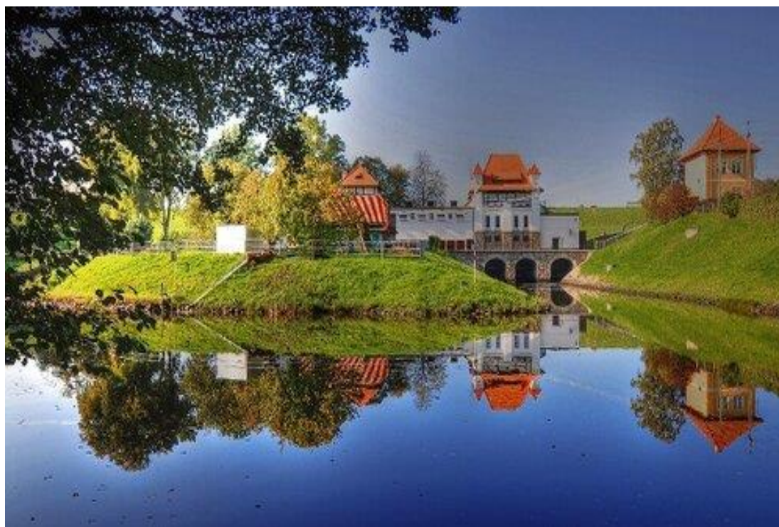
Straszyn hydro plant
