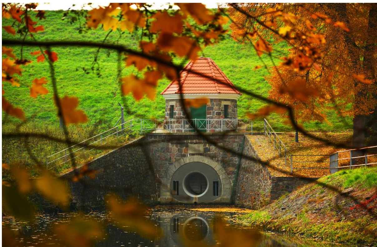
Straszyn hydro plant
