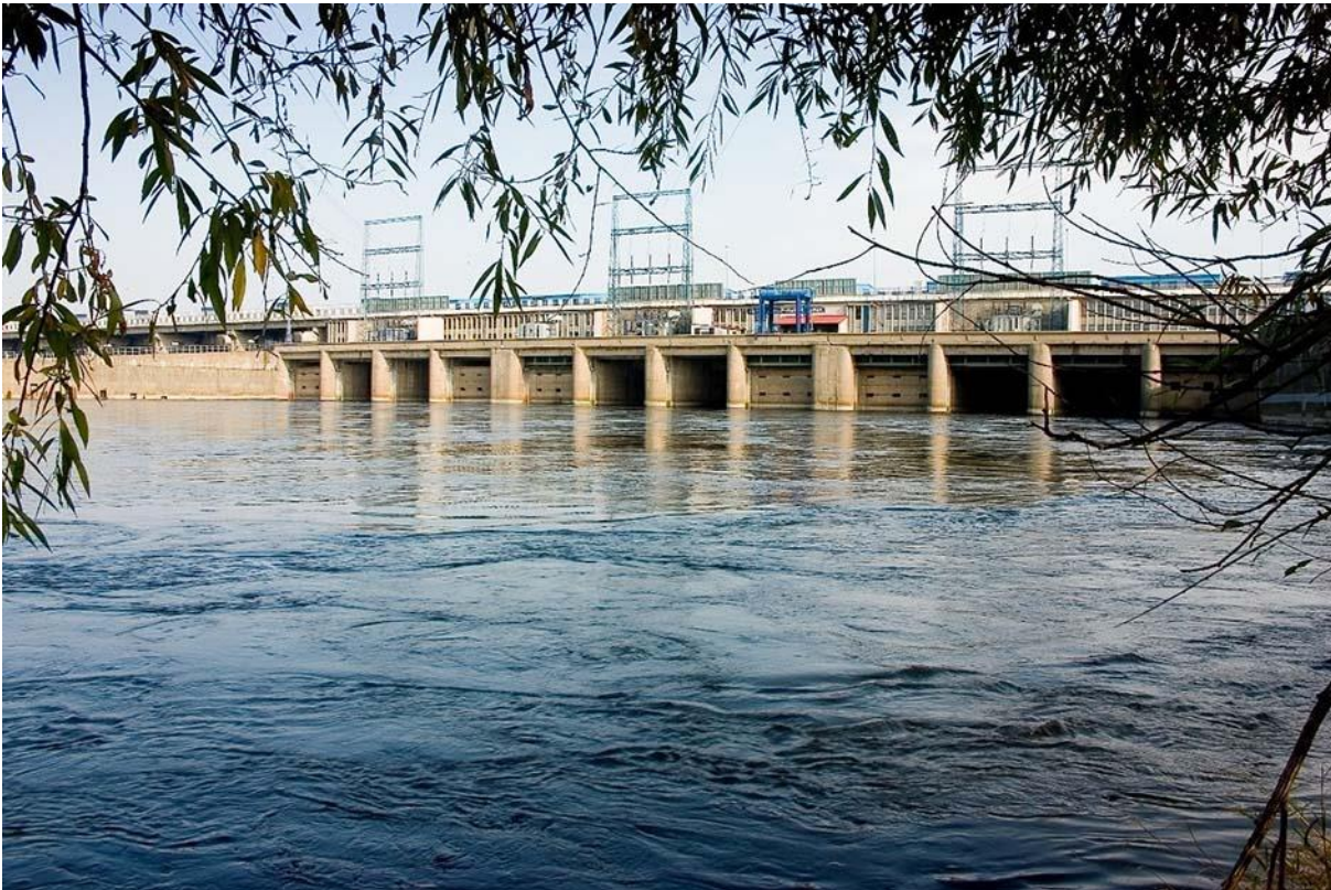
Włocławek Hydroelectric Power Station
