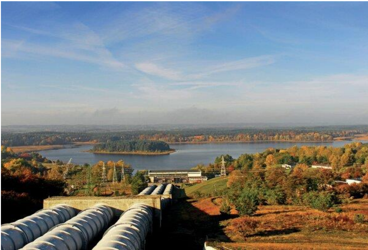
Pumped-storage power plant Żydowo
