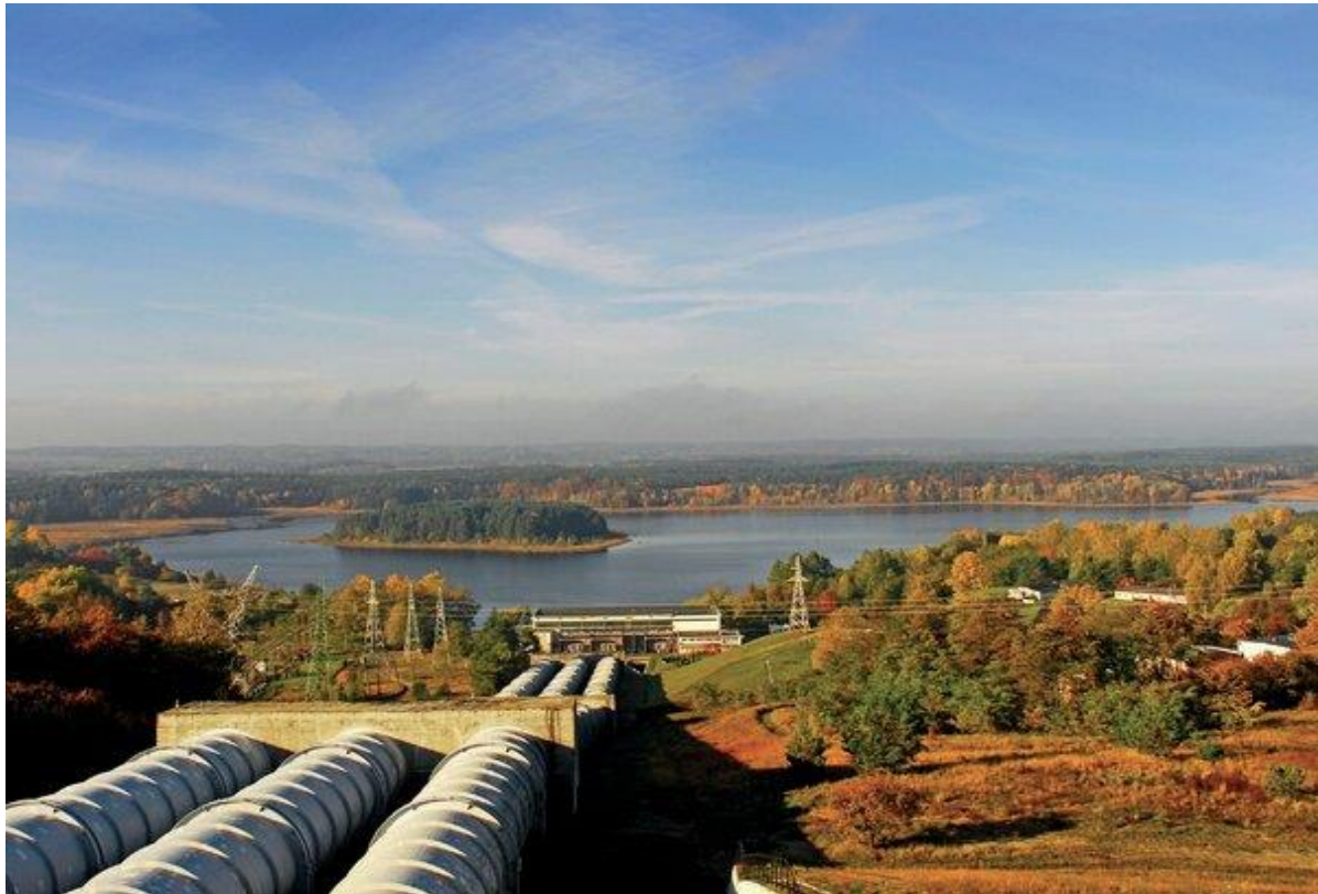
Pumped-storage power plant Żydowo
