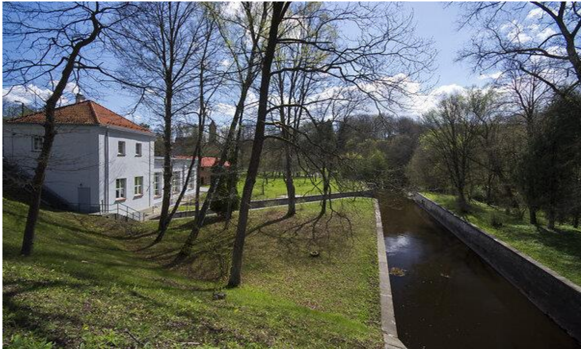
Pieniężno hydro plant
