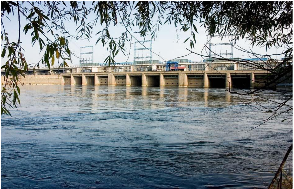
Włocławek Hydroelectric Power Station
