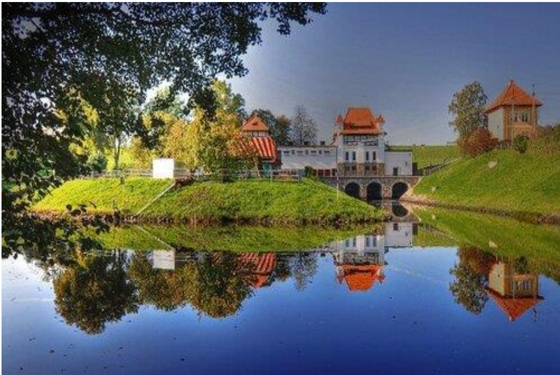
Straszyn hydro plant
