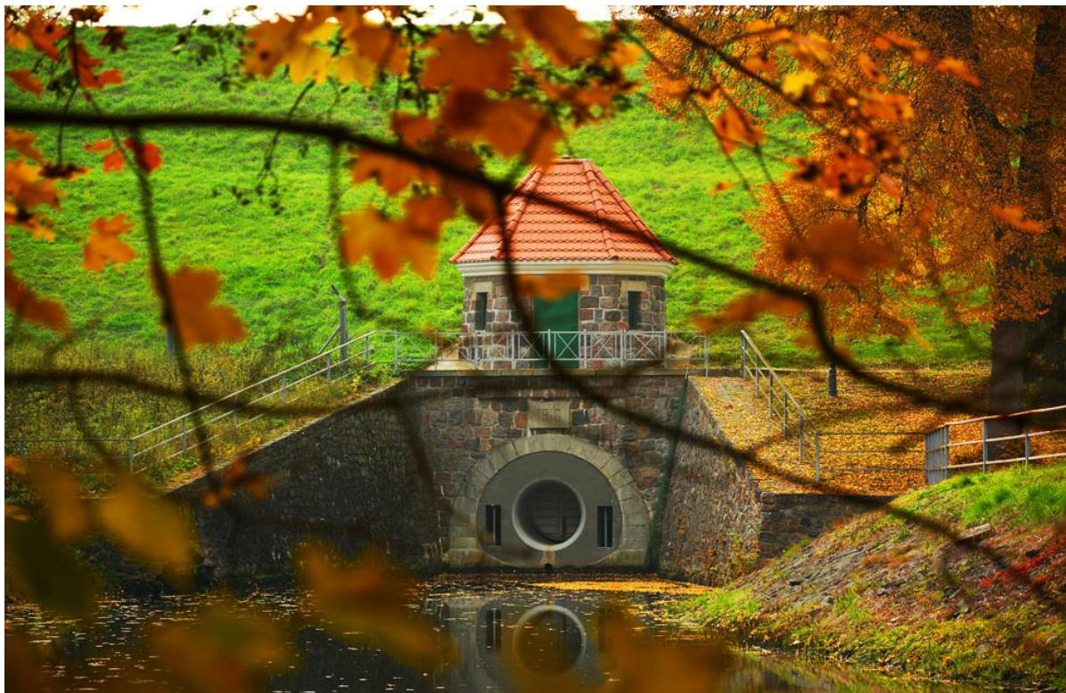
Straszyn hydro plant
