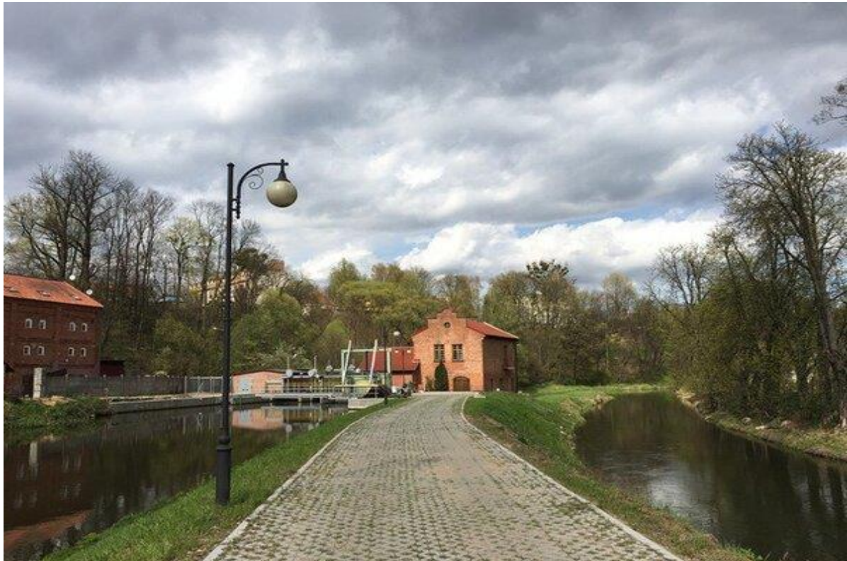
Lidzbark Hydro plant
