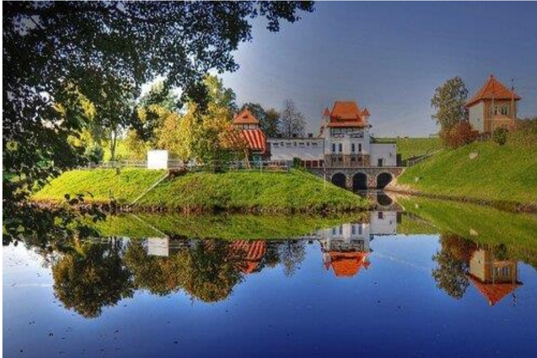
Straszyn hydro plant
