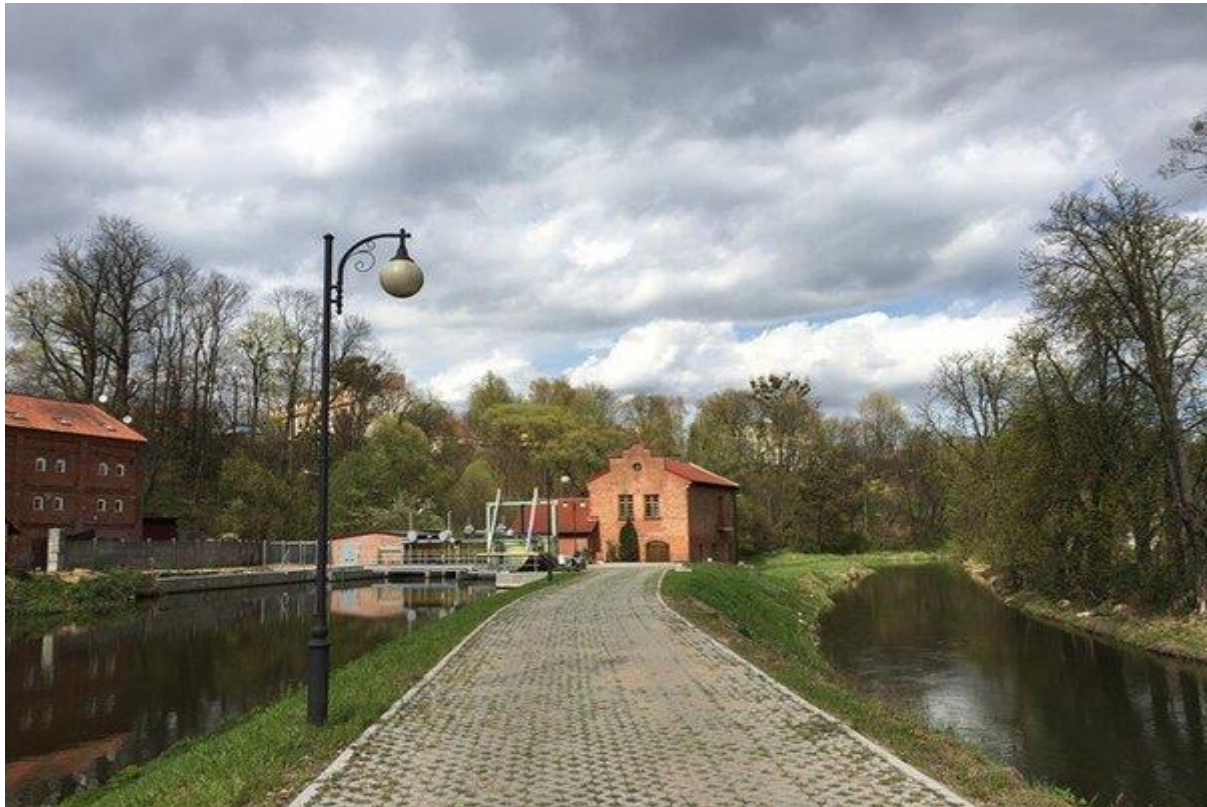
Lidzbark Hydro plant
