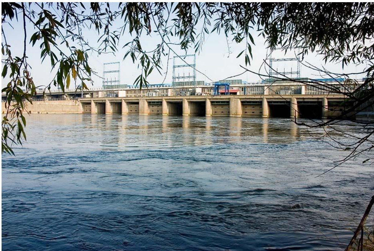
Włocławek Hydroelectric Power Station
