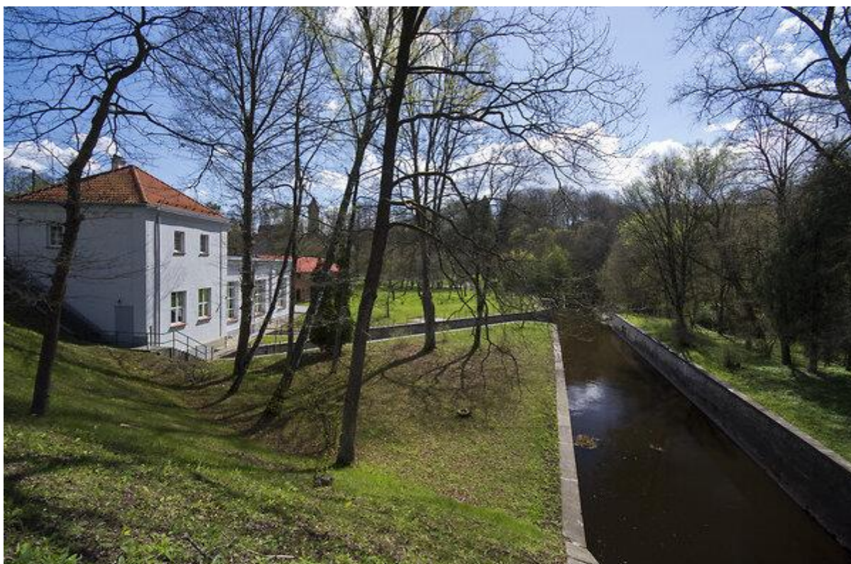
Pieniężno hydro plant
