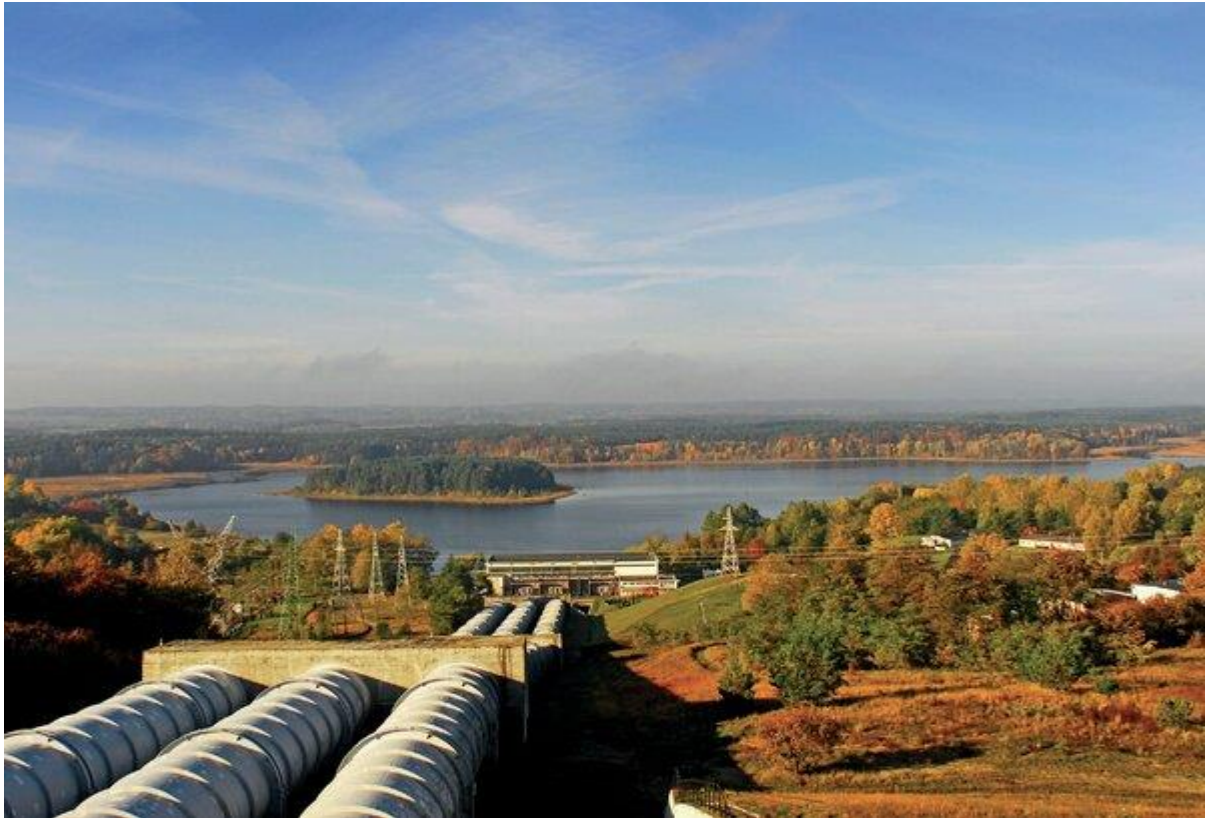
Pumped-storage power plant Żydowo
