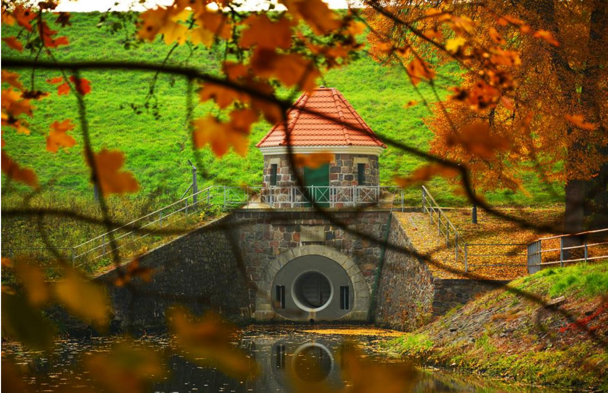
Straszyn hydro plant
