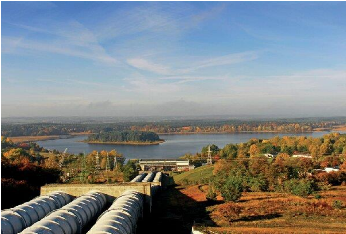
Żydowo pumped storage power plant
