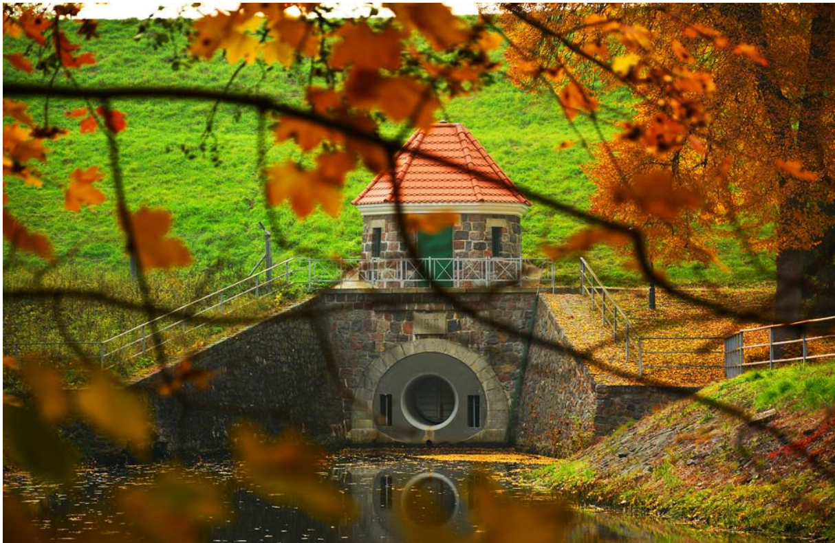
Hydro plant in Straszyn
