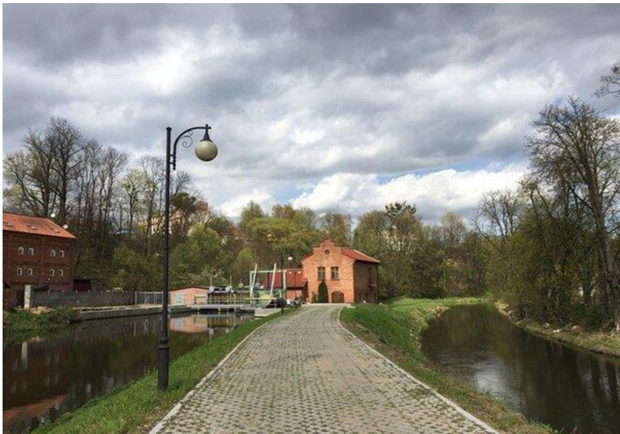
Hydro plant in Lidzbark
