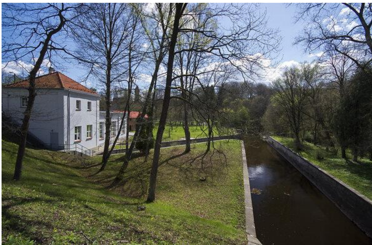
Hydro plant in Pieniężno
