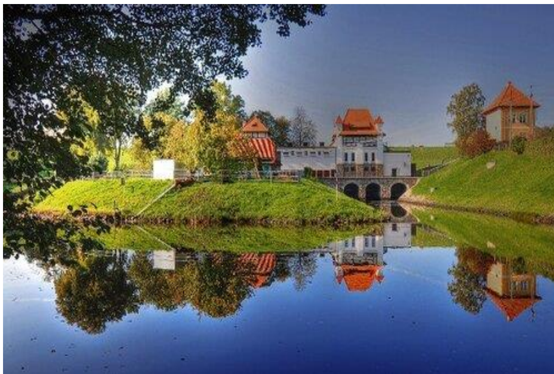
Hydro plant in Straszyn
