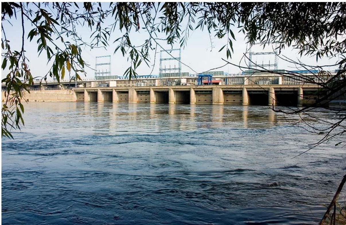
Włocławek Hydroelectric Power Station
